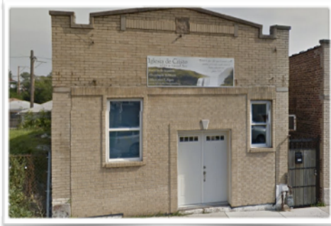
Church Building in Grand Ave
